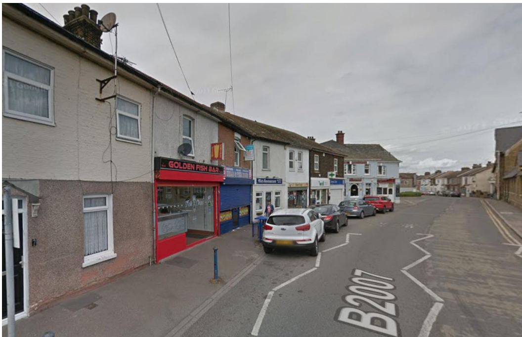
View of Railway Terrace
